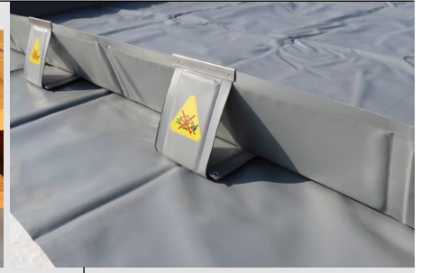
Detail of lateral reinforcements
