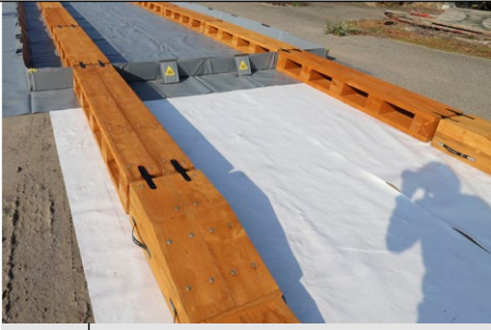
Pool with wooden ramps
