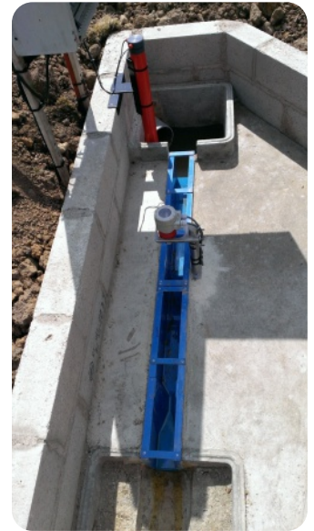
Example of installation with civil engineering
